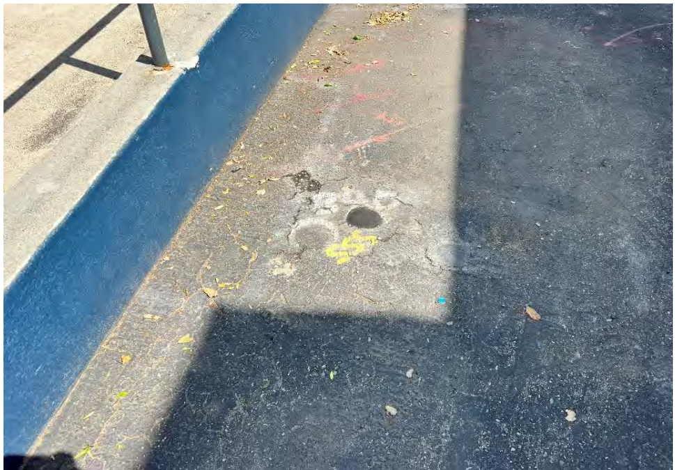
Photograph 4: View of backfilled and patched original and co-located boring for B40.
