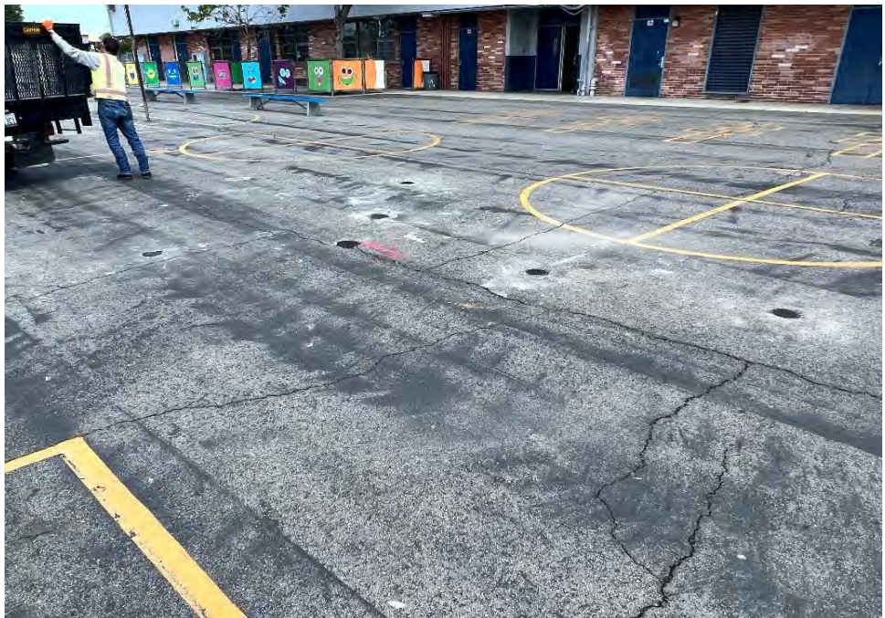
Photograph 6: View of backfilled and patched step-out locations for the original boring B34.
