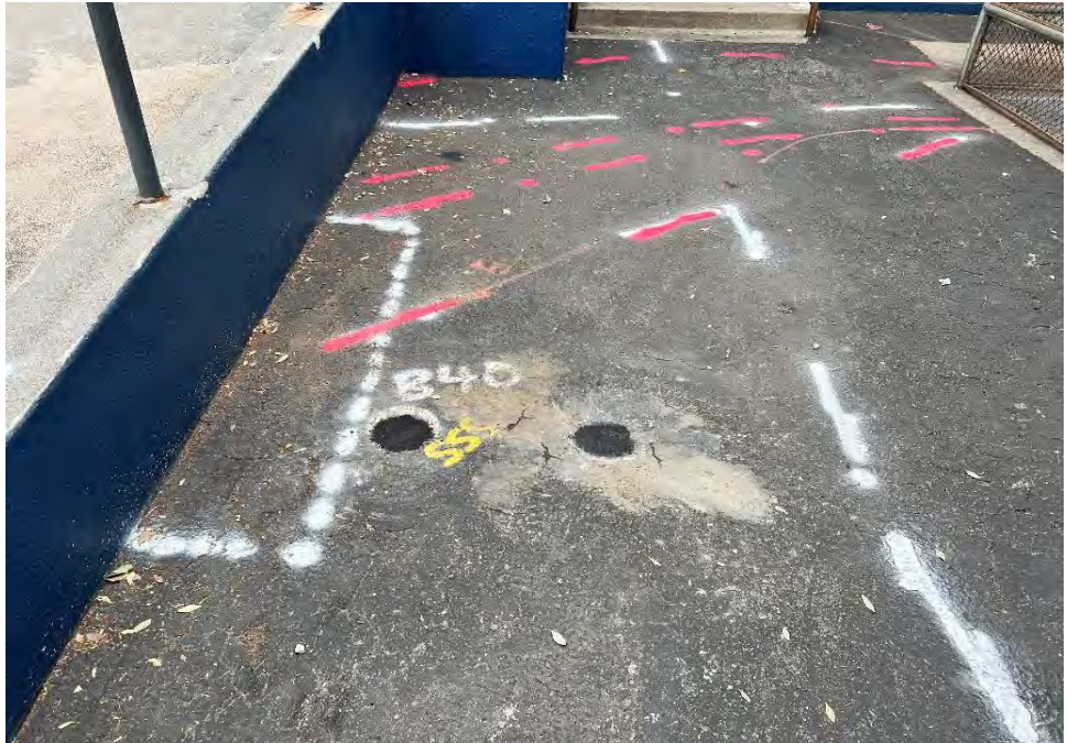
Photograph 5: View of a typical backfilled and patched borings on-site.
